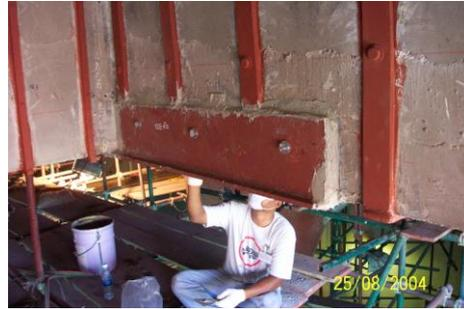
Figure 13: Strengthening of beam (a) Slot in beams (b) Beam after strengthened
